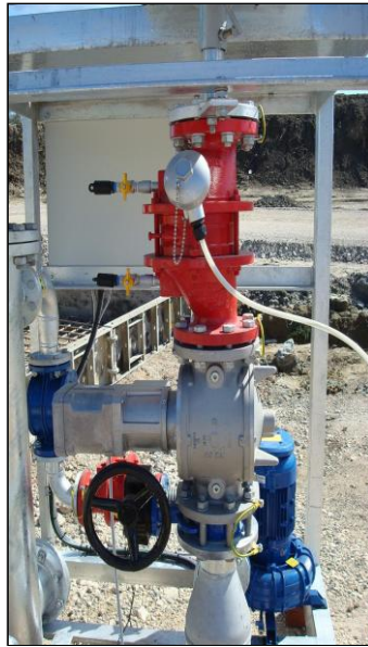
Flame Arrester electric operated safety shut-off valve
